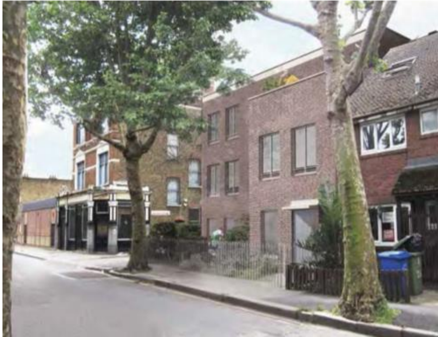
View of Block A from Braganza Street with the Royal British Legion building beyond
